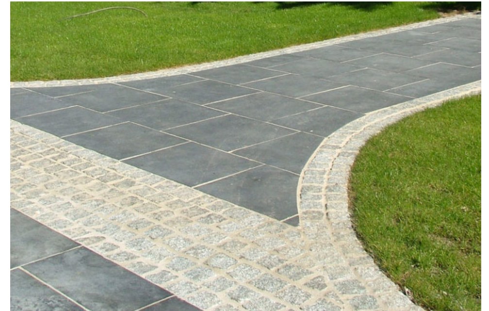
Proposed: use of local materials to create aesthetically pleasant and well designed pathways. Consider of cobbles/textured grain to edges and thresholds.
