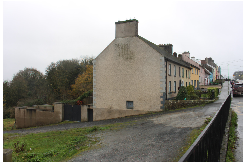
Kingscourt - existing: unattractive building wall lacking art installation.
