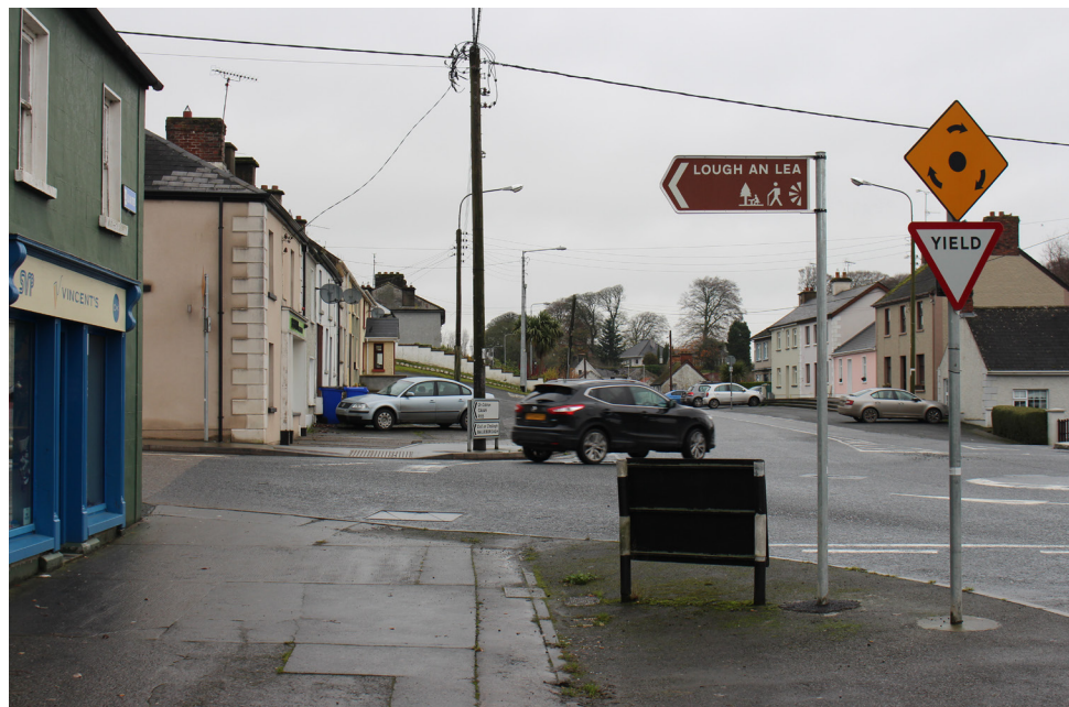
Kingscourt - existing: paved area that does not add to the streetscape aesthetics neither provide amenities for the residents.
