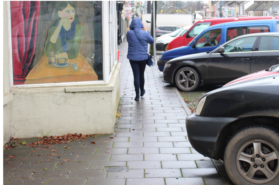
Kingscourt - existing: narrow pavements with poor quality surface and cars invading it.
