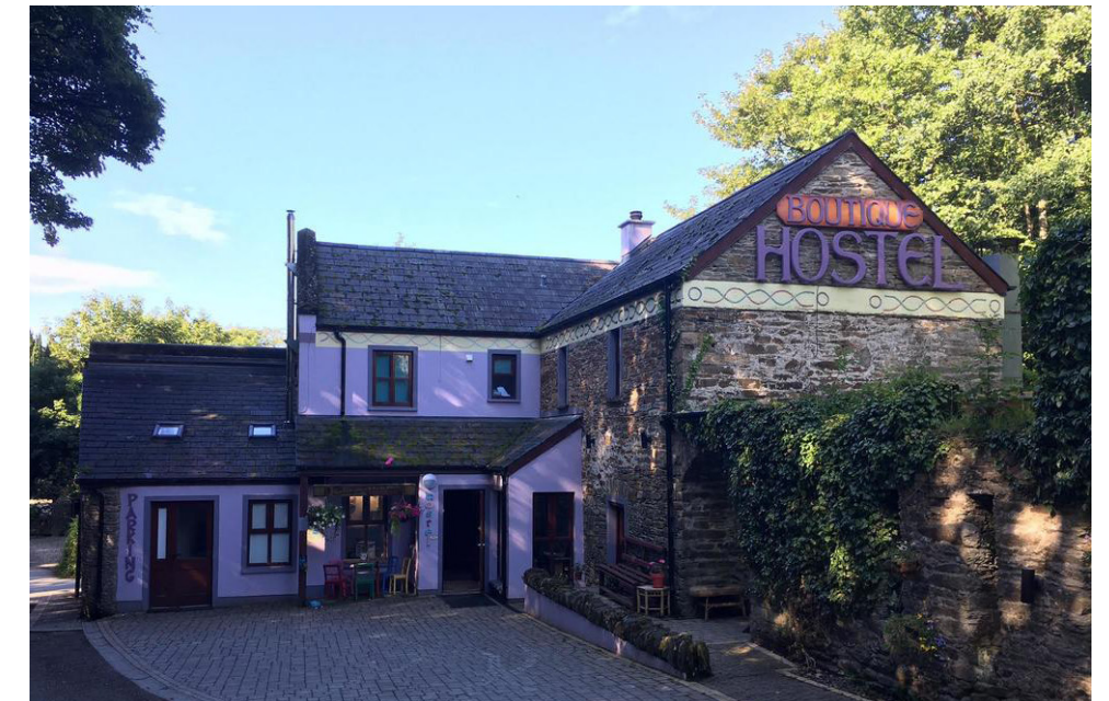
Proposed: example of sensitive redevelopment of a historic site that preserves its heritage significance.
