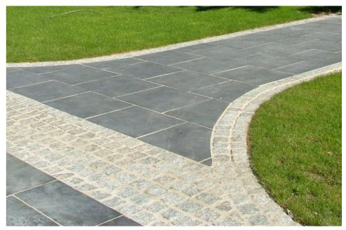
*Proposed: use of local materials to create aesthetically pleasant and well designed pathways. Consider application of cobbles/textured grain to edges and thresholds.*
