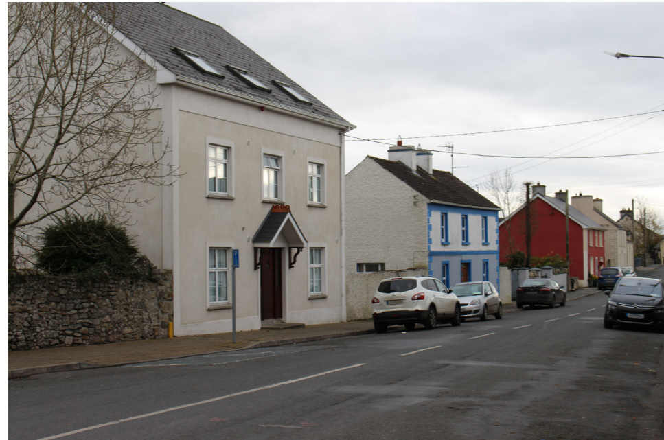
Lough Gowna - existing: key façades in need of refreshment
