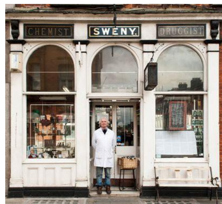
Opportunity to restore the vernacular atmosphere of Dowra through traditional landscape practices and the restoration of buildings
