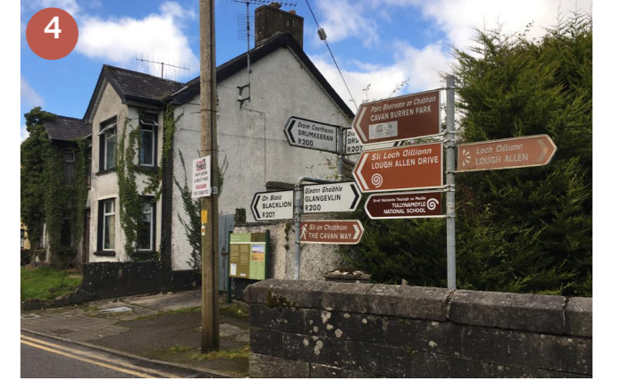
Modern signage detrimental to the vernacular atmosphere of the village
