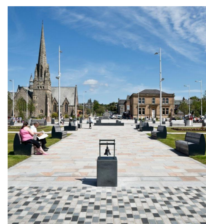
Stone paving to replace concrete
