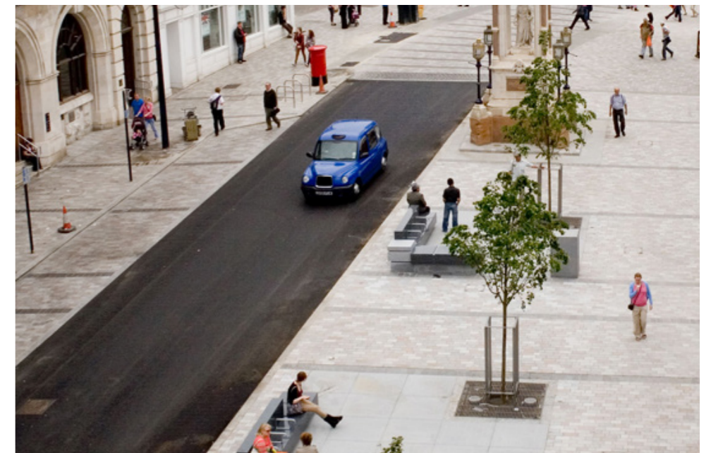
Proposed: convert two-ways carriageway into a one-way traffic lane to calm traffic and allow for wider pavements.
