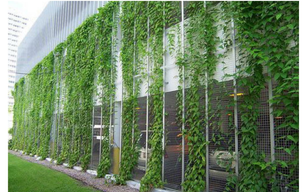
Proposed: screening of the premises through climbing vegetation and aesthetically pleasant fencing.
