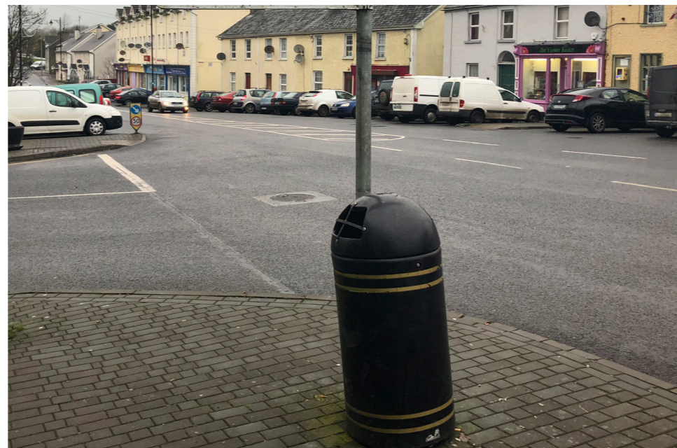
Ballyjamesduff - existing damaged waste bins - no allowance for recycling.
