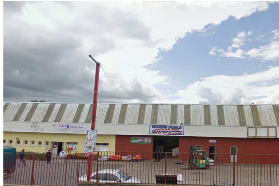
Ballyjamesduff - existing: views over industrial premises on approach road to town.
