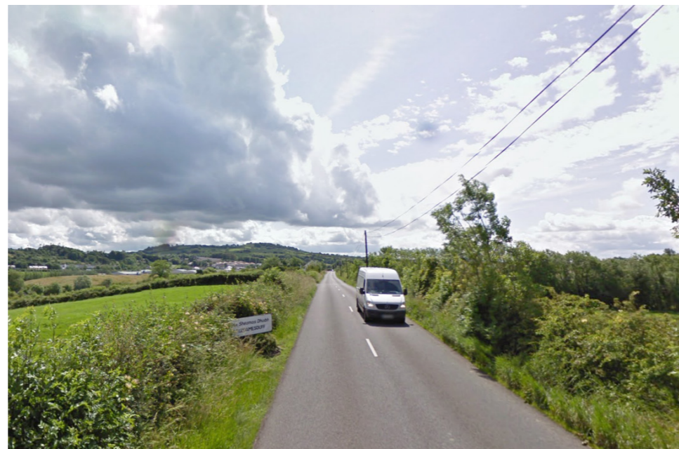
Ballyjamesduff - existing: a lack welcoming approach signs.
