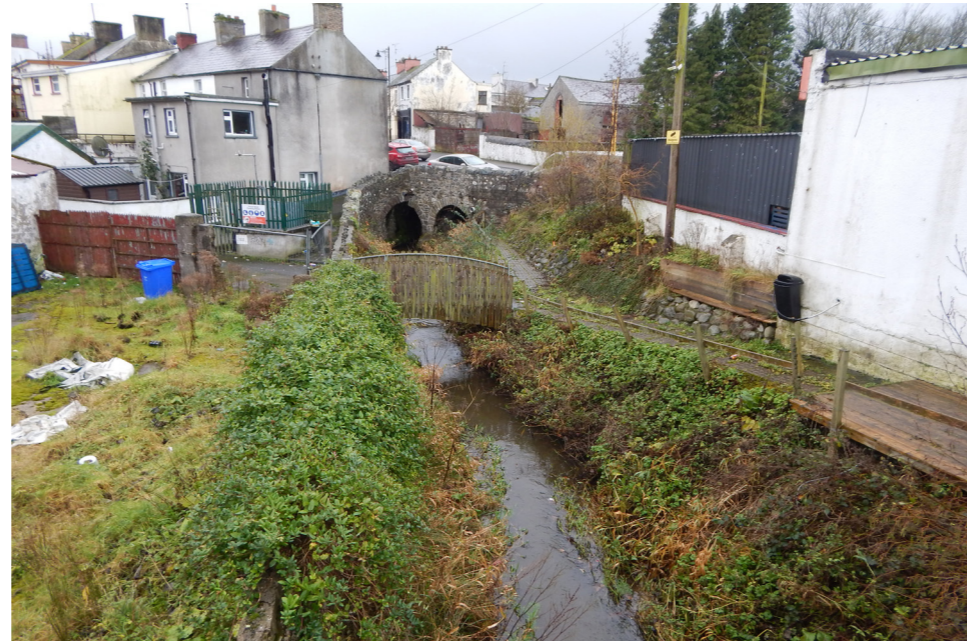
Ballyjamesduff - existing: unsightly views over the river and adjacent plots.
