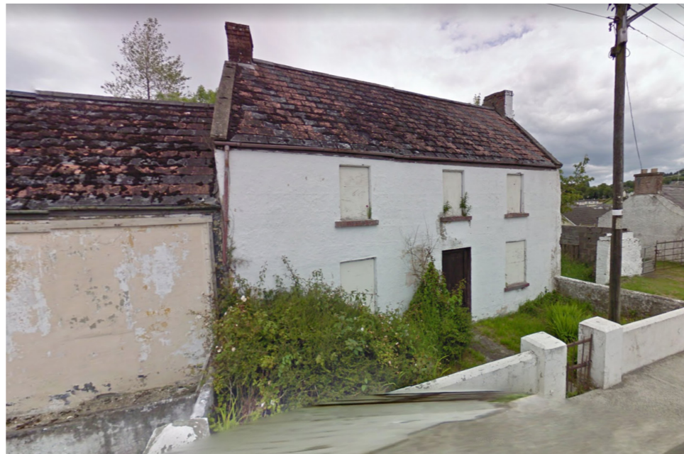
Ballyjamesduff - existing: derelict and abandoned properties along Cavan Road
