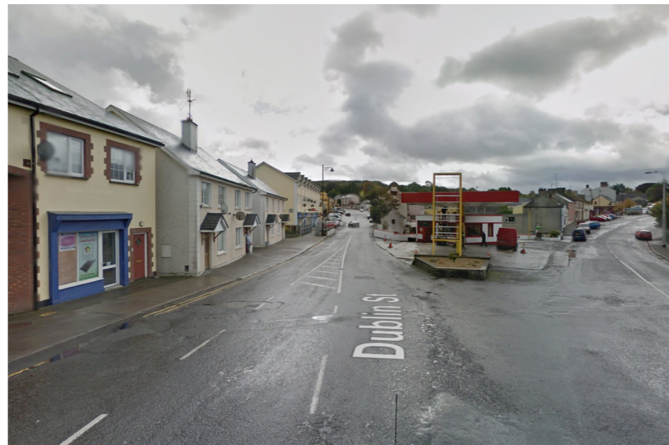
Ballyjamesduff - existing: junction between Market Street, Cavan Road and Dublin Road.
