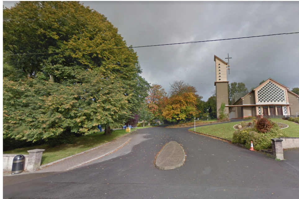
Ballyjamesduff - existing: the approach road to County Cavan Museum lacks character and is poorly signed
