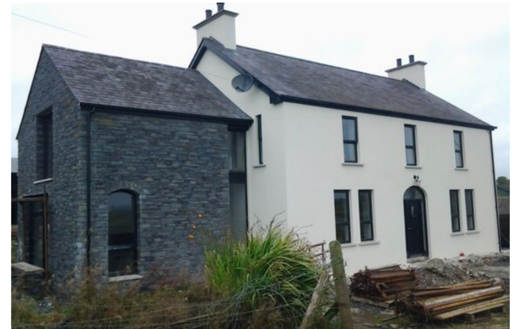
Proposed: sensitive redevelopment of derelict properties, adding a contemporary twist to historic built forms.
