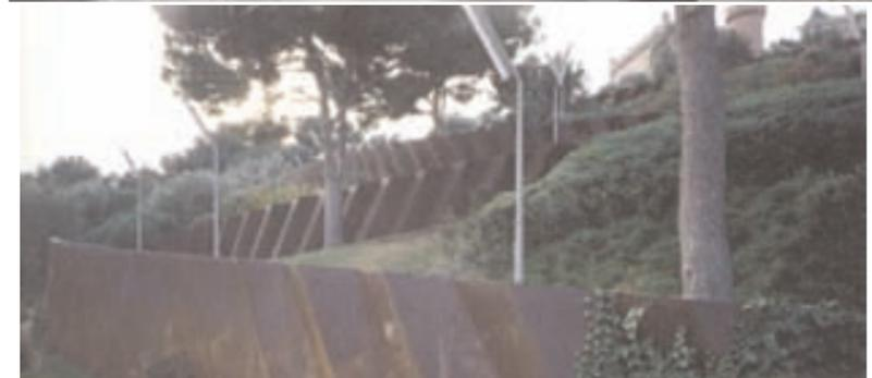
to negotiate the slope the ramps climb in a zig-zag on walls constructed to contain the levelled ground
