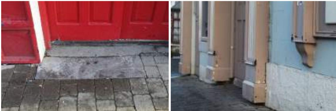
Fig 7. Former threshold in front of The Whistle Stop Bar indicating the location and size of former door openings and Fig 8. Steps removed outside The Riverfront Hotel resulting in the architraves and pilaster not meeting the footpath surface.
