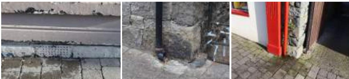
Fig 27. Subfloor vent, Fig 28. Cast-iron rainwater downpipe and Fig 29. Downpipe at footpath surface
