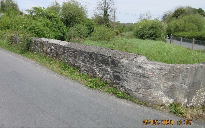
Fig. 9: East parapet wall of bridge, with concrete wing wall to corner
