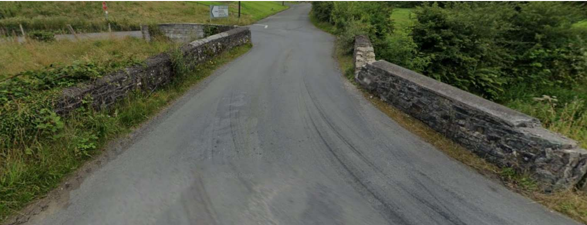
Fig. 11: Deck of bridge, view southeast (Google maps)
