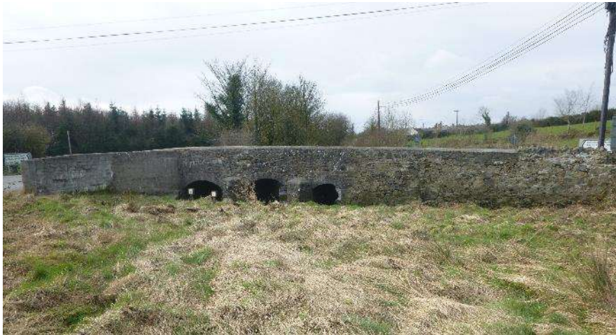
Fig. 3: Upriver elevation of the bridge
