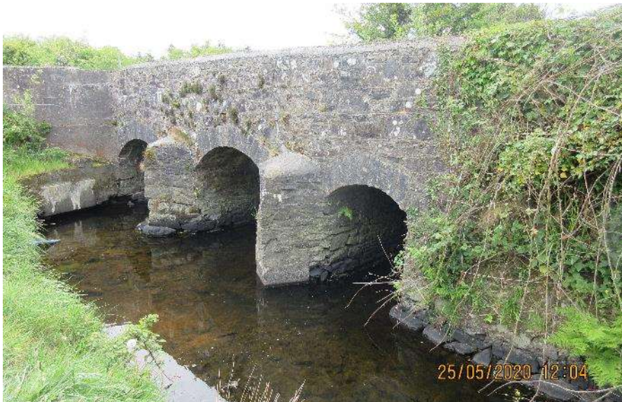
Fig. 4: The three arches and cutwaters, upriver elevation of the bridge
