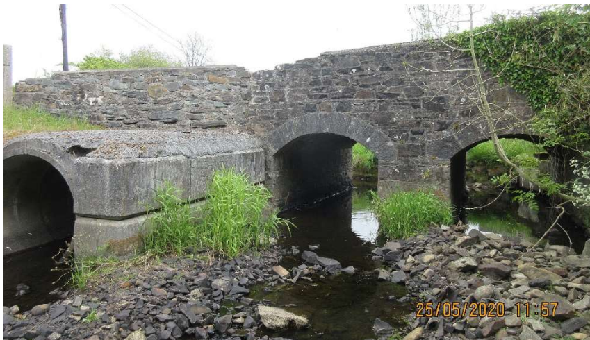
Fig. 7: Downriver elevation of the bridge, showing concrete pipe and embankment constructed to the westernmost arch of this elevation, obscuring original cut stone arch.
