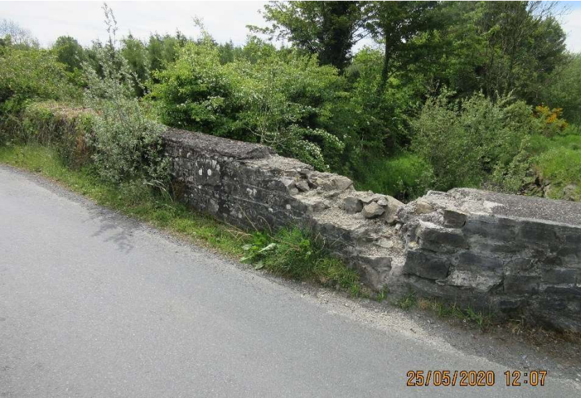
Fig. 10: West parapet wall, showing collision damage to stonework
