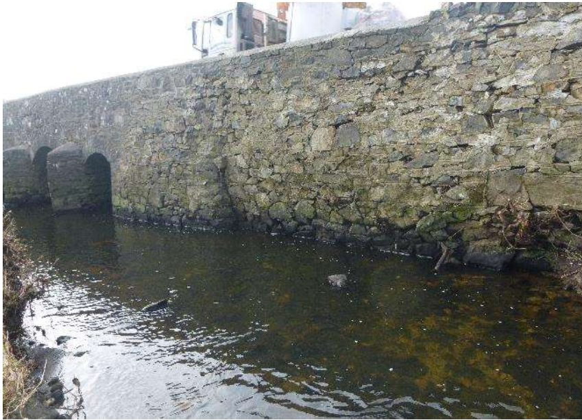
Fig. 6: Upriver elevation of the bridge and wing wall, showing the course of the river as it approaches from northwest.
