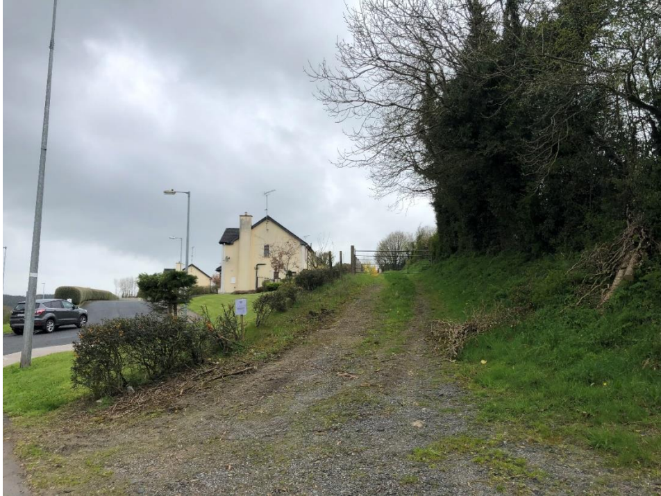
Fig 1.5 Existing Junction to the R188 Cootehill-Cavan Road along the Errigal route to be upgraded to facilitate proposed cycle / pedestrian route. Proposed timber gate staggered junction and signage to be provided for traffic safety reasons.
