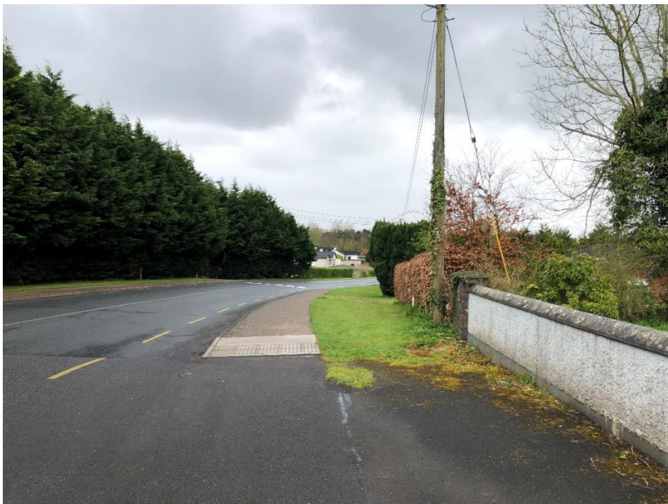
Fig 1.5 Existing Junction to the R188 Cootehill-Cavan Road along the Errigal route to be upgraded to facilitate proposed cycle / pedestrian route. Proposed timber gate staggered junction and signage to be provided for traffic safety reasons.
