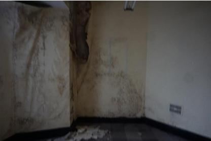
Photograph 71 – View of water damage at ground floor level
