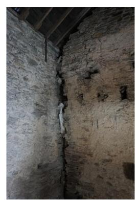
Photograph 17 - Internal View of the sheds to be deconstructed. Internal walls in disrepair and cracking occurring. (Shed 2)
