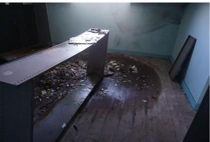
Photograph 52 - Image of water ingress on the top floor
