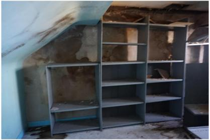
Photograph 53 - View of damage occurring due to water ingress
