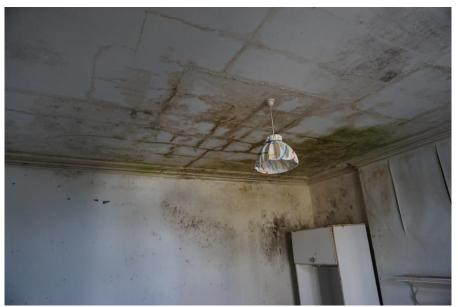
Photograph 59 – View of water ingress damage
