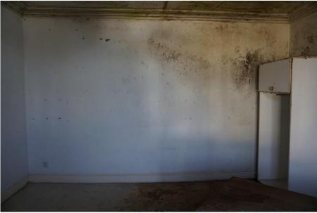
Photograph 58 – View of the room with water ingress damage
