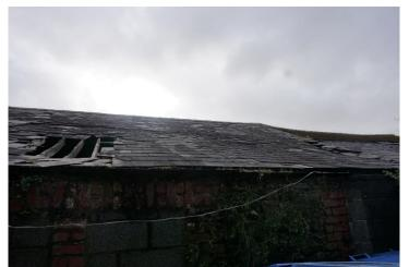
Photograph 8 – View of rear outbuilding. Natural slate finish, some slates missing and slipping.
