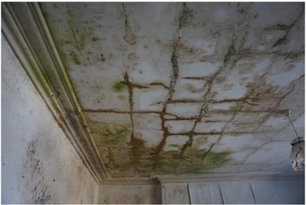
Photograph 57 - View of damage to the ceiling due to water ingress
