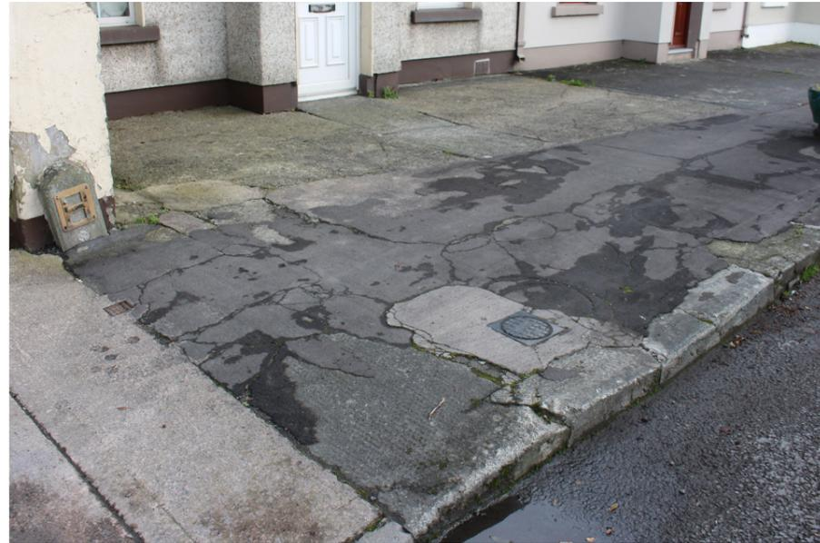
Cootehill - existing: uneven paving littered with chewing gum and current design enables parked cars to overlap the kerb.
