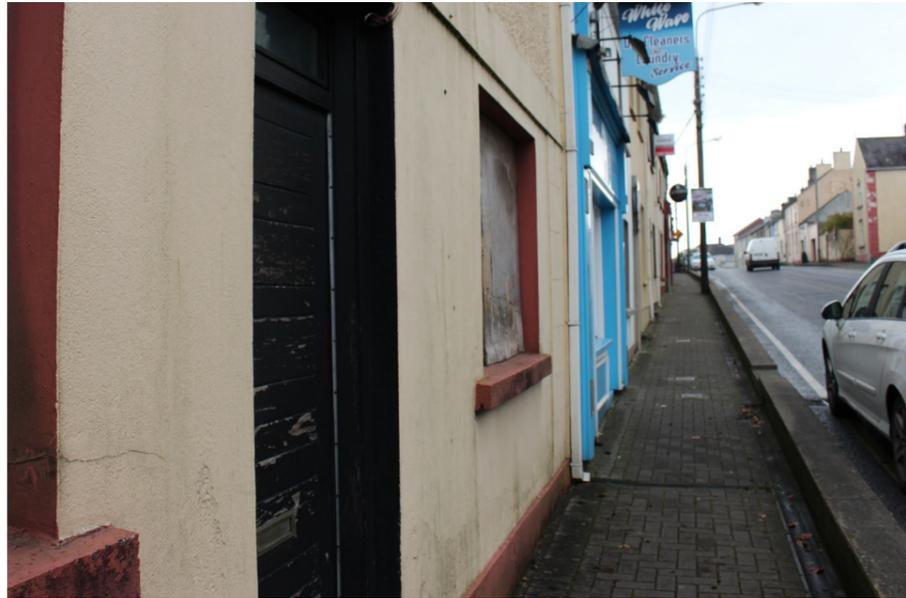
*Belturbet - existing: narrow and uneven paving of poor quality.*
