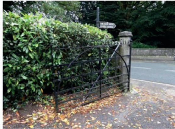
A series of vehicular and pedestrian gates are located along the stone walls, affording access to the church grounds. The gateways are constructed in either cut -stone or from course rubble and have wrought-iron gates..
