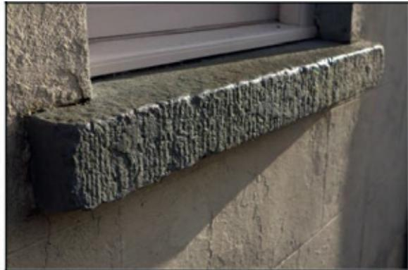
Detail of tooling on window sill
