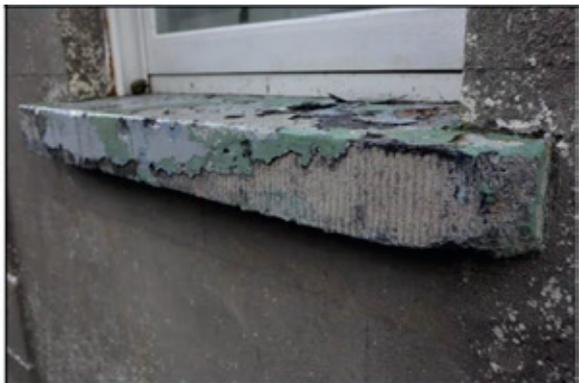
Tooling marks on stone threshold and window sill
