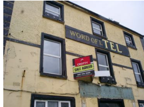
Intact PVC windows on front elevation
