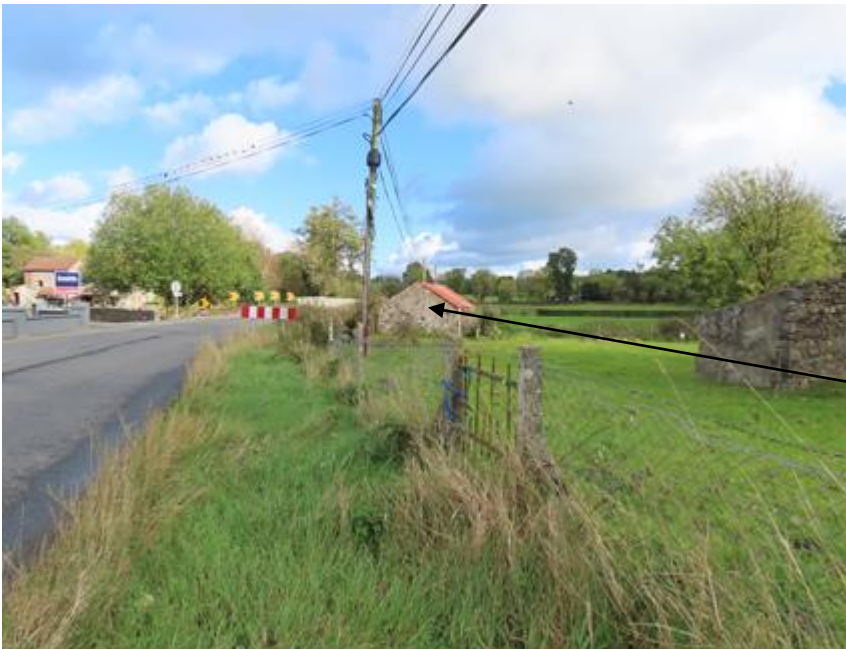
Photo 1 – looking north east towards Derrylea Bridge. Small stone shed to be demolished is indicated
