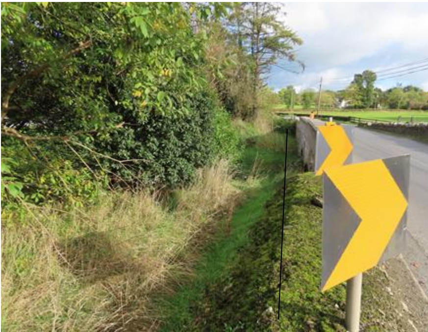
Photo 3 – position of proposed walkway to north of bridge structure
