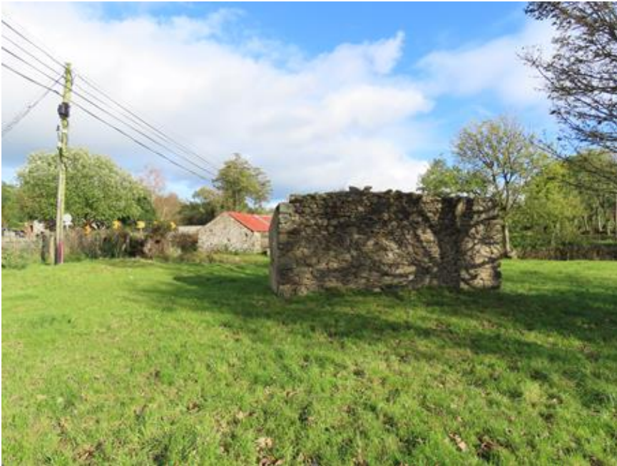
Photo 17 – Two stone buildings on western downstream side of river
