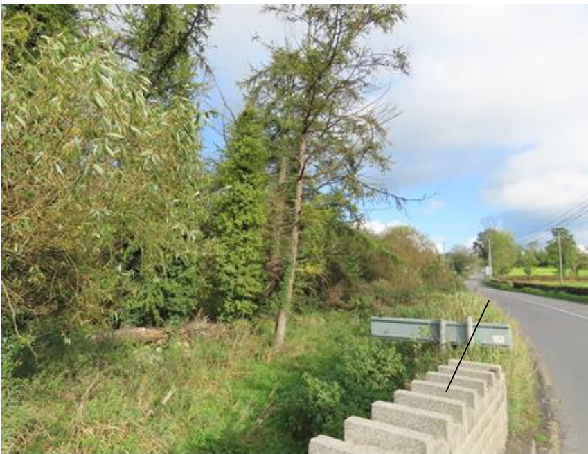
Photo 5 – eastern side of bridge – location of proposed walkway indicated
