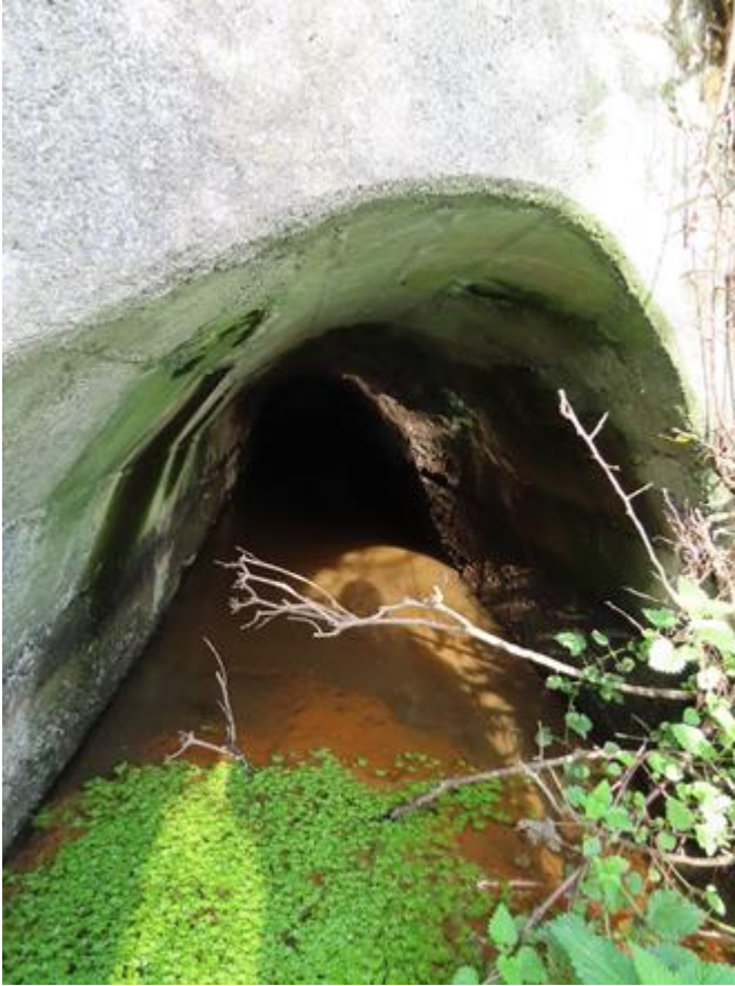
Photo 22 - Smaller arch which originally carried the mill race
