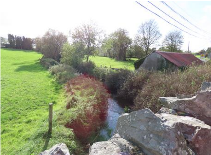
Photo 15 – watercourse downstream of bridge
