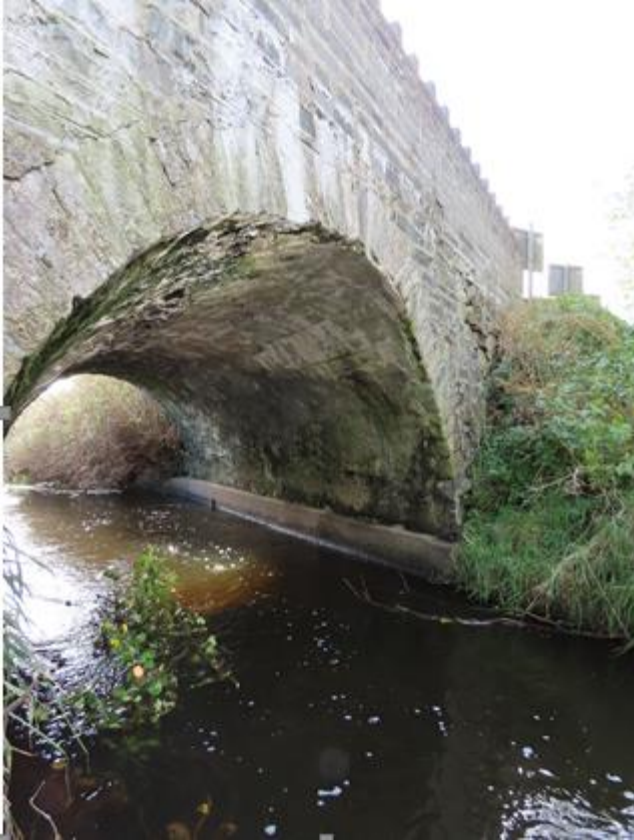
Photo 12 – grout and shuttered concrete sealing the undersurface of the western arch
