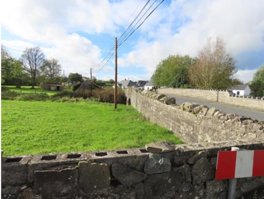
Photo 8 – looking west towards downstream face of bridge
