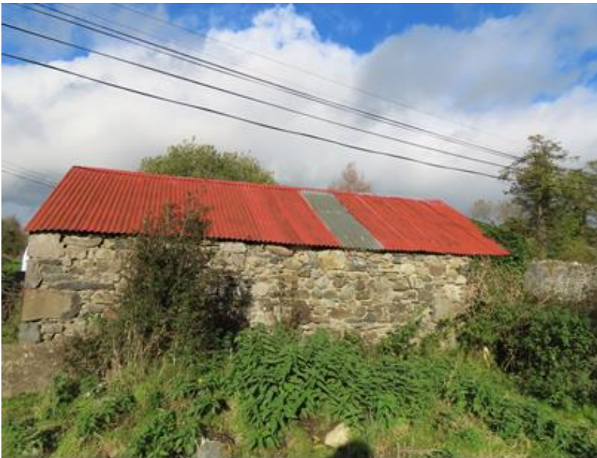
Photo 19 – rear of farm shed with thick stone walls
