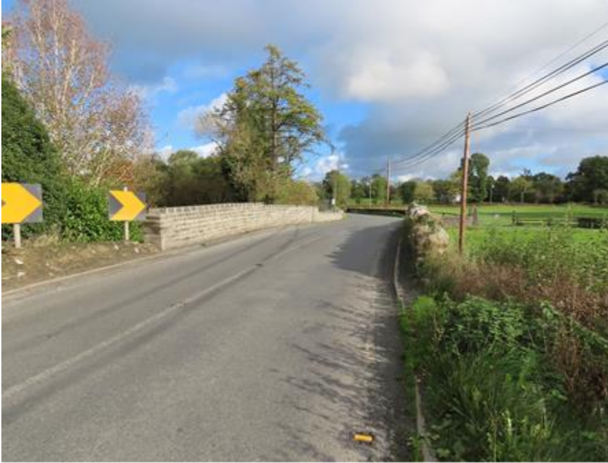
Photo 2 – looking east across Derrylea Bridge
