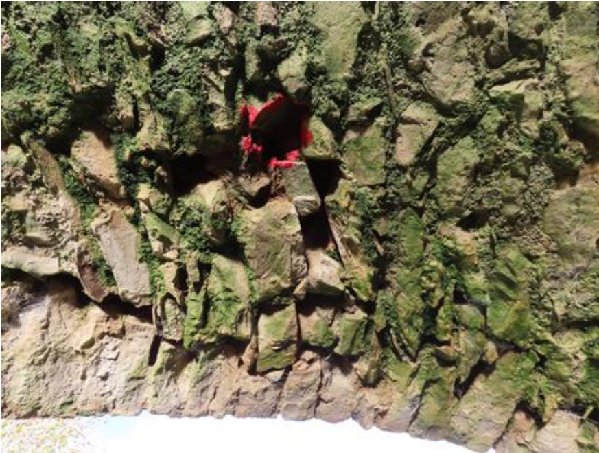
Photo 11 – crevice marked for retention for bats close to upstream face of eastern arch
