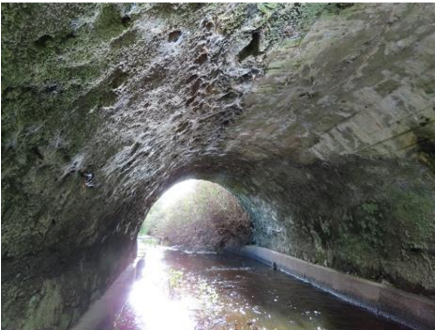
Photo 13 – grout and shuttered concrete sealing the undersurface of the western arch
