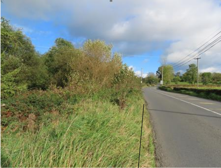
Photo 6 – eastern side of bridge – position of proposed walkway
