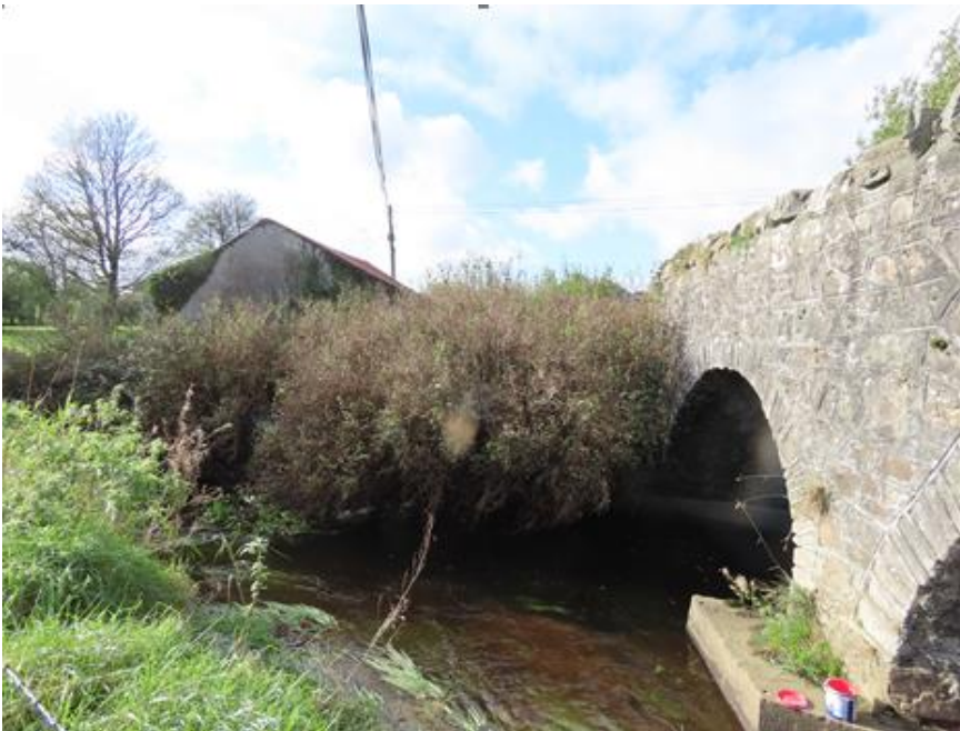
Photo 9 – downstream face of bridge
