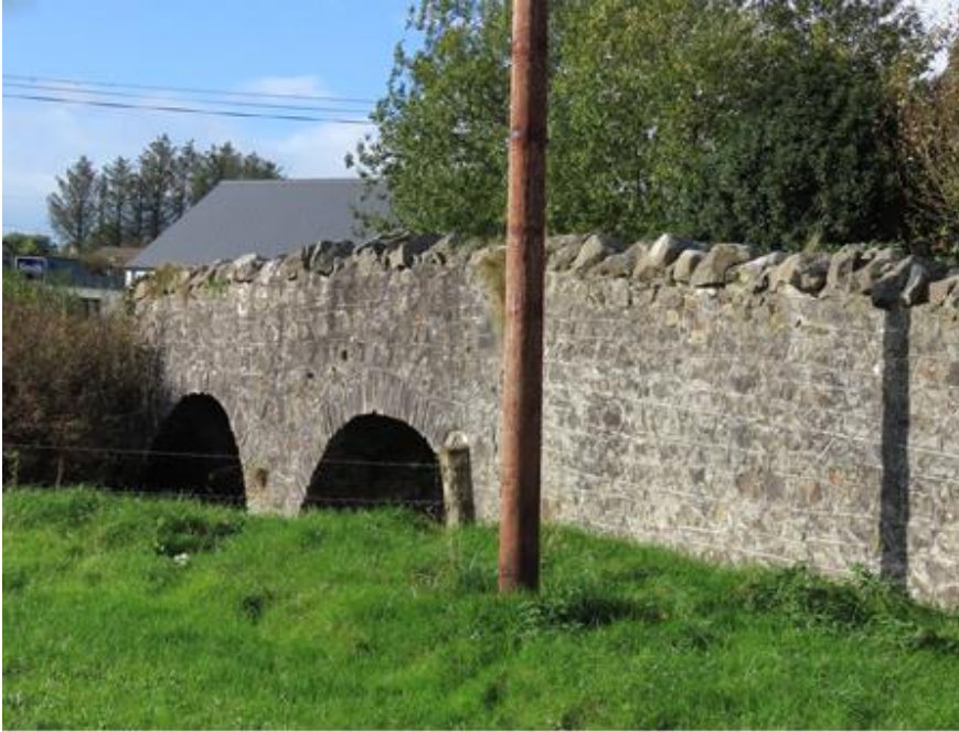
Photo 14 – downstream elevation of bridge
