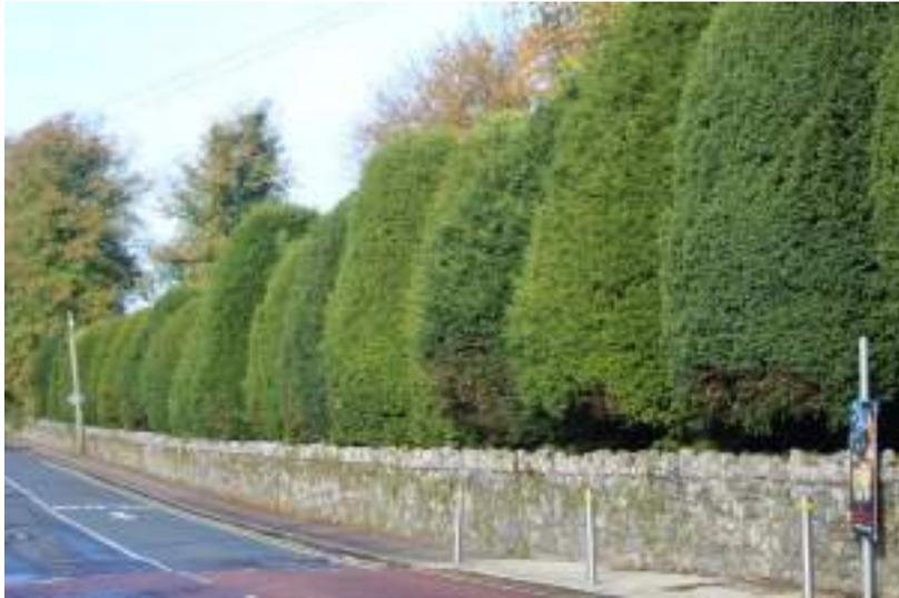
Fig 22. Rubble stone boundary wall to St. Lurgan’s Church
