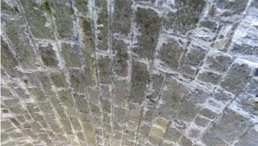
**Photo 13** – view of stonework under eastern arch which has been well-grouted in the past
