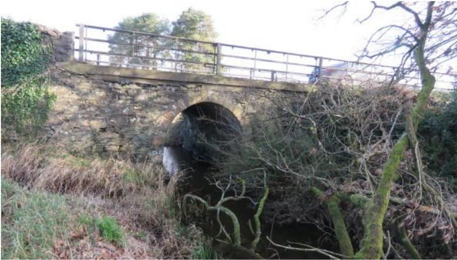
**Photo 3** – southern face of western arch. A large oak tree stands just downstream of the bridge. Some boughs have broken and have fallen into the river causing a blockage.
