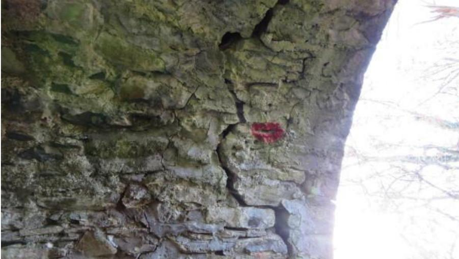
**Photo 9** – Crevice marked for retention for bats towards southern face of western arch
