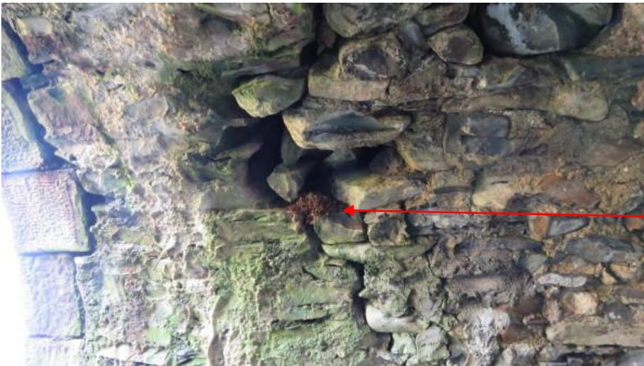
**Photo 6** – void in stonework close to northern face of western arch with remains of dipper's nest
