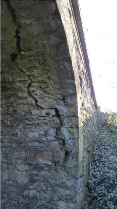
**Photo 5** – deep fissure running around arch barrel 0.5 – 1m in from southern face of western arch
