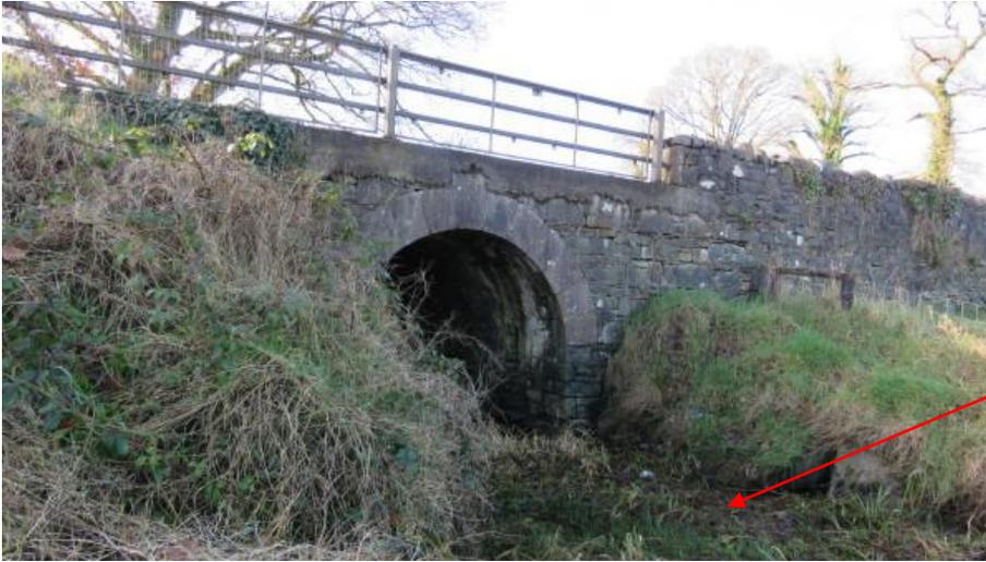
**Photo 11** – northern face of western arch. The channel upstream of this arch is blocked with vegetation which should be removed.
