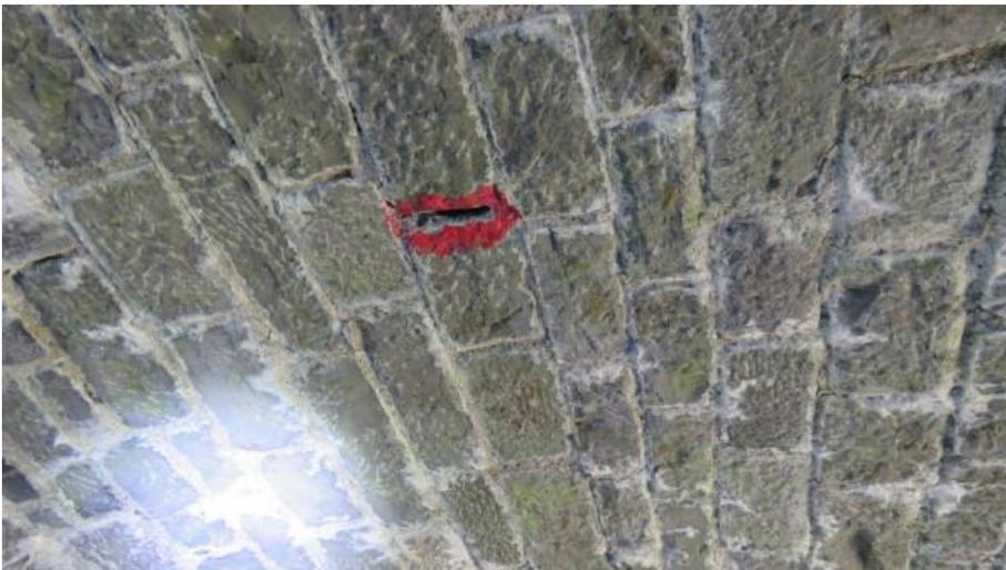
**Photo 16** – Crevice marked for retention for bats in stonework at apex of eastern arch
