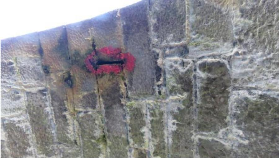
**Photo 15** – Crevice marked for retention for bats behind upstream facing stones of eastern arch
