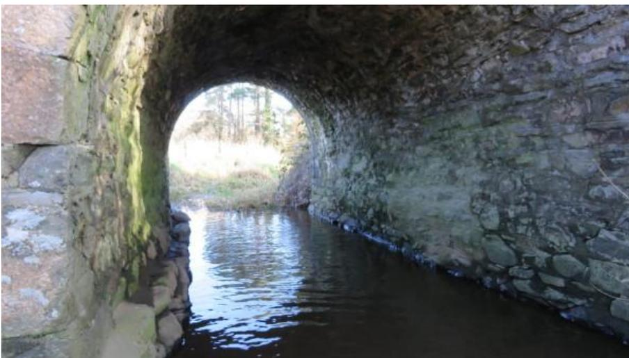
**Photo 4** – view under western arch. There is a narrow plinth of stone running along the base of the western abutment.
