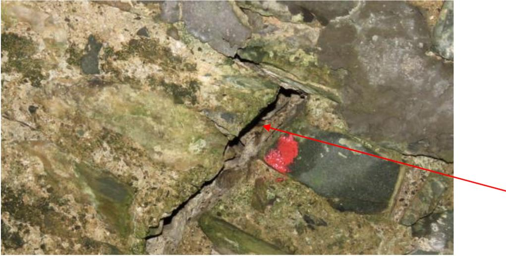
**Photo 7** – crack midway under western arch with evidence of bat usage in the form of staining
