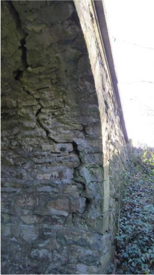
**Photo 5** – deep fissure running around arch barrel 0.5 – 1m in from southern face of western arch
