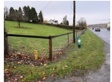
Above Before and after on the N3 at Poles
