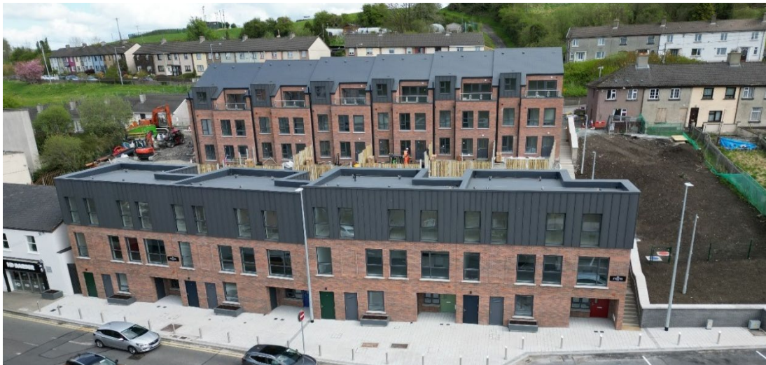
St. Brigid's Terrace, Cavan – Phase 1
