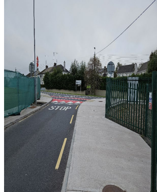
Above: Completed Junction Works
