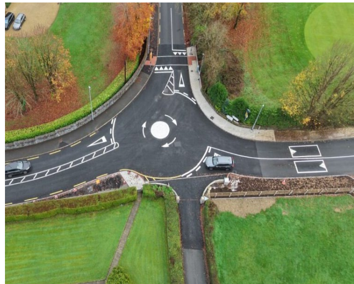
Above Completed Roundabout Works
