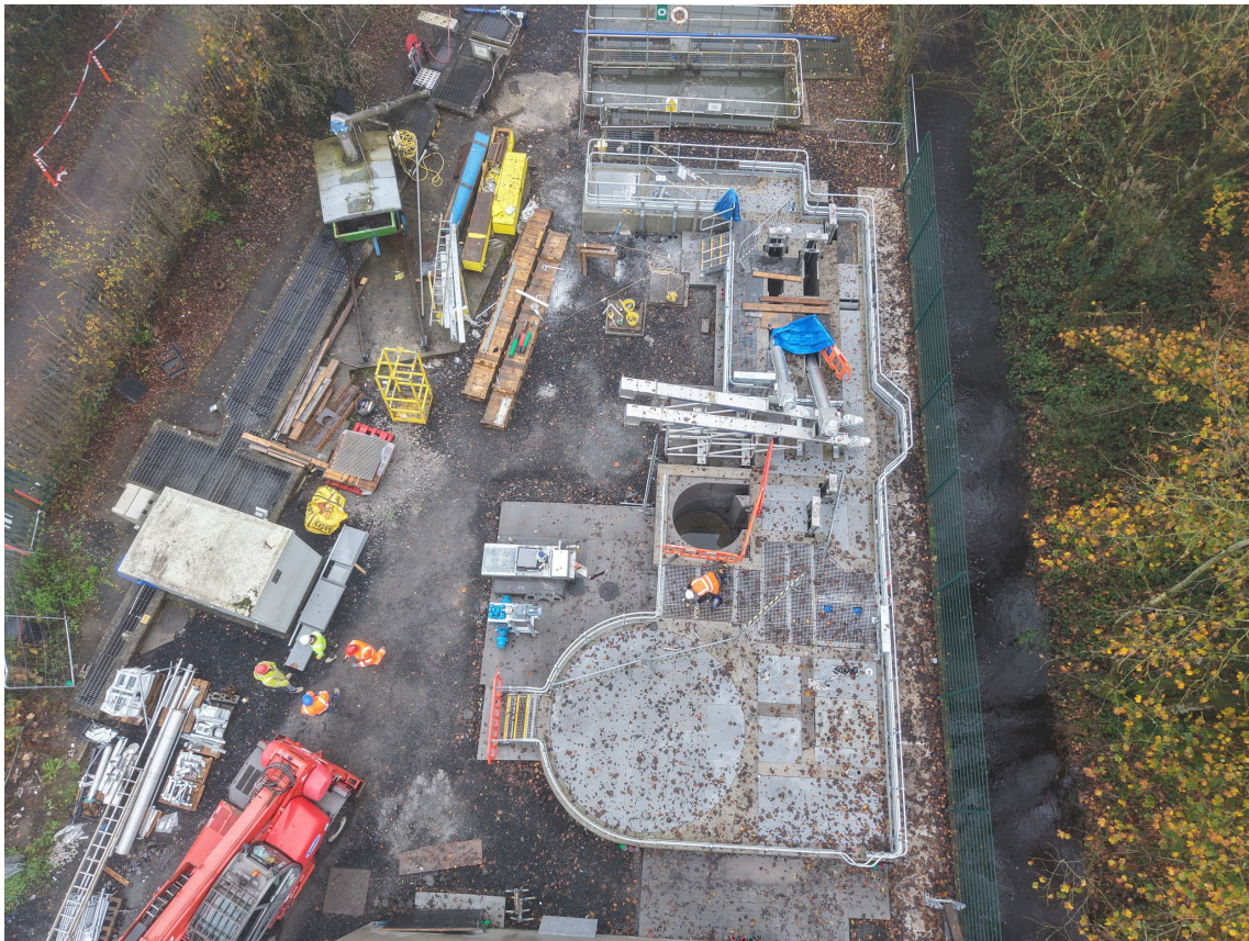
Decking at Inlet & Grease Chamber
