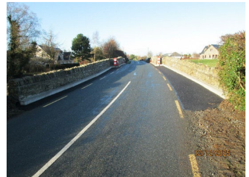
Above: Mullagh Bridge Before and After works
