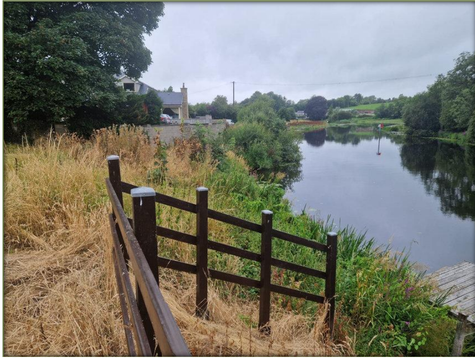
Figure 9e – Looking East / Upstream of the River
