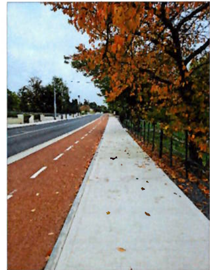
Above: Complete Phase 1 Works
