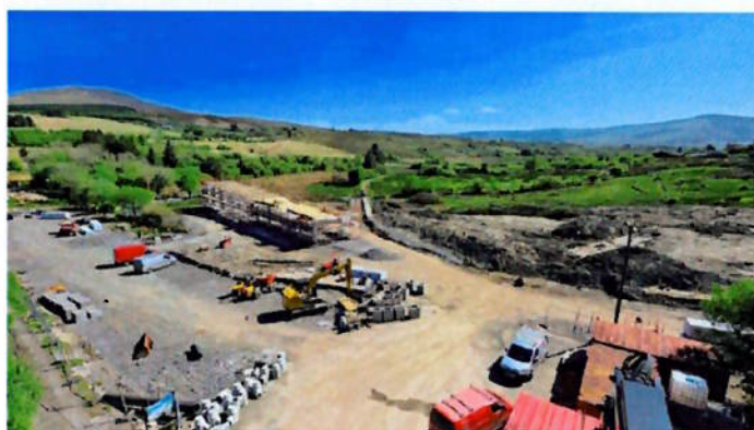
Shannon Pot Construction Site
