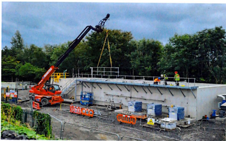
Works ongoing on site Upgraded Ballyjamesduff Wastewater Treatment Plant Virginia WWTP
