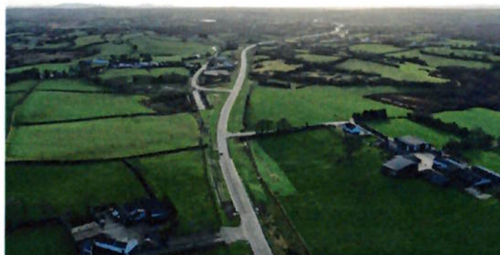
Left: View of completed Bridge 3 in the townlands of Ballytrust Lower and Legwee
