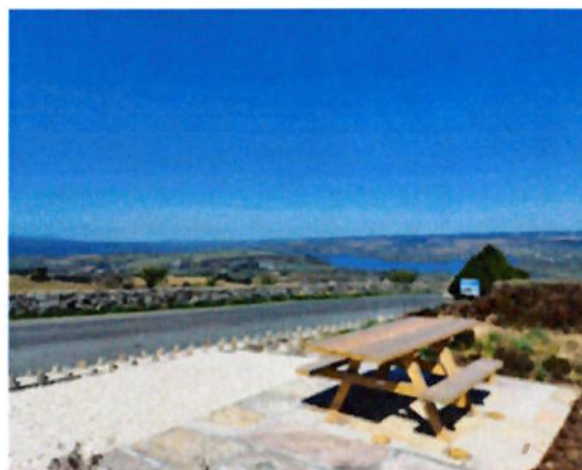
Cornagee Viewpoint Upgrade Works
