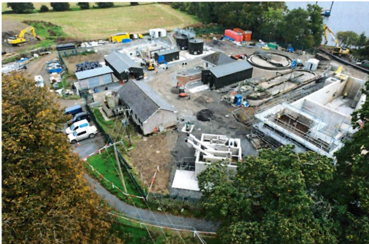
Aerial View showing progress to date on site of Upgraded Virginia Wastewater Treatment Plant
