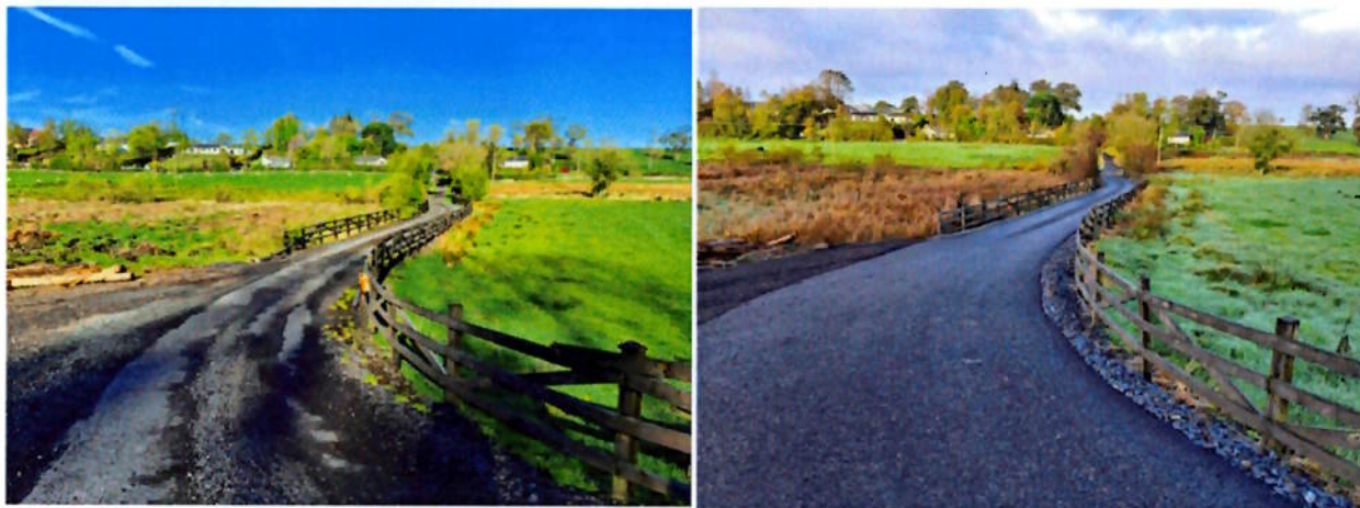
Above: LIS works at Tonymore before and after
