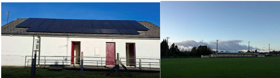
Installation of 13.5 Kw Solar System (PV Panels) at Denn GAA and Upgraded FL500W LED around the lower pitch
