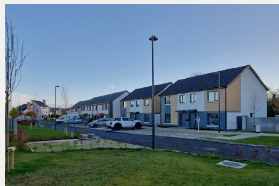
Boreen Bradach, Kinnegad 12-unit scheme, delivered by Westmeath County Council as part of the Accelerated Delivery Programme
