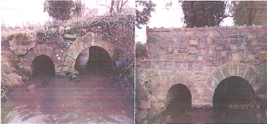
Keadew Bridge - Before and After
