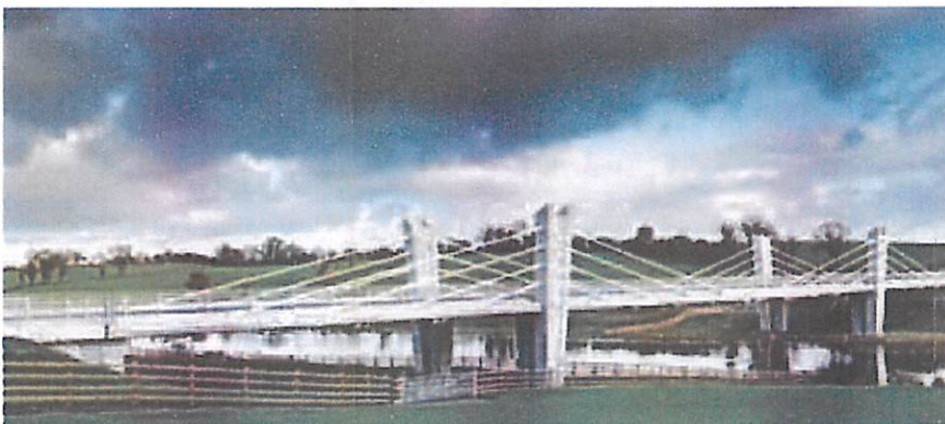
Extradosed Type Bridge over the River Erne
