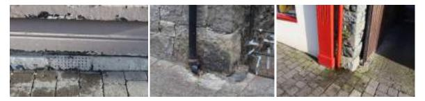
Fig 27. Subfloor vent, Fig 28. Cast-iron rainwater downpipe and Fig 29. Downpipe at footpath surface
