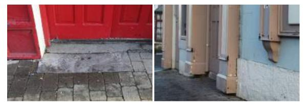
Fig 7. Former threshold in front of The Whistle Stop Bar indicating the location and size of former door openings and Fig 8. Steps removed outside The Riverfront Hotel resulting in the architraves and pilaster not meeting the footpath surface.
